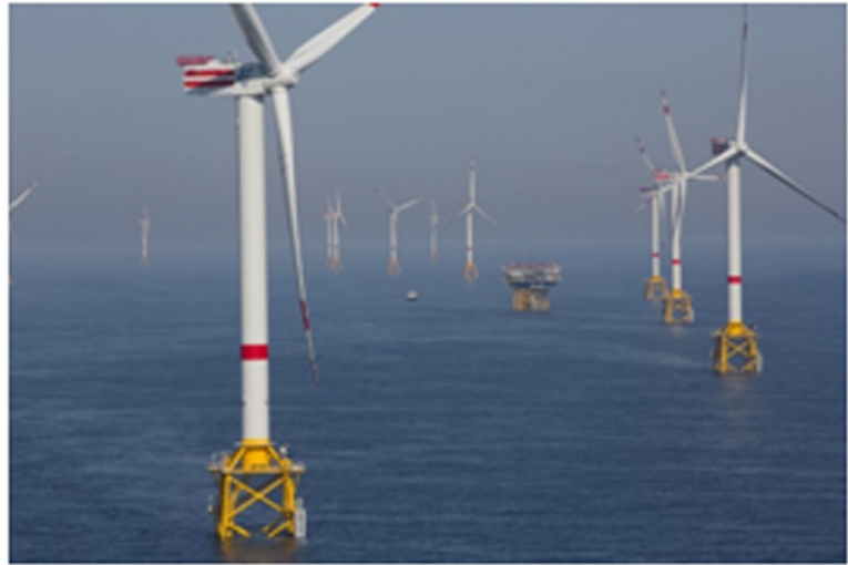
*C-power wind farm in Thornton Bank
